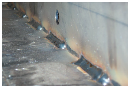
Concave weld seam grinding
