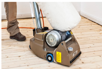
Refurnishment of wooden floors | Sleeve sander
