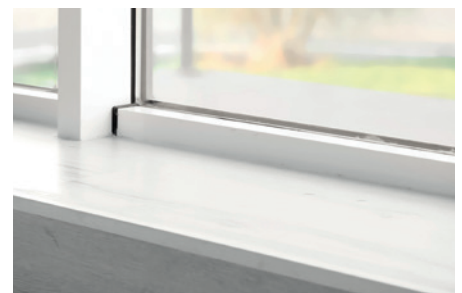
Granite window sills and steps | Sanding of cutting edges
