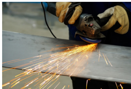
Trimming of steel plates for welding
